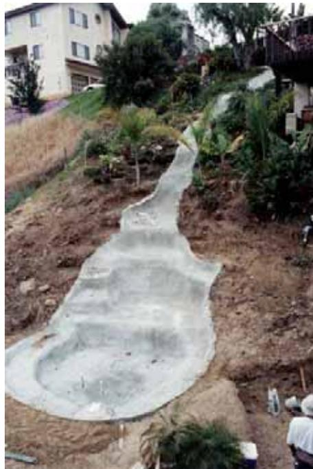
properties were in line, down the side of the mountain. The waterfall started in the back yard of the first house continued to a pond at the bottom house, 135 feet below. Because of the position of the crane, the crane operator and the placement crew were unable to see each other and use hand signals. So we used 2-way radios with hands-free head sets. Believe me, craning over a house is not that big a deal!
