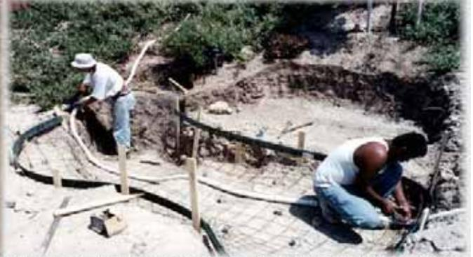
Dobie blocks are used to hold the rebar off the ground so the concrete will totally encase it. Also, flexible PVC pipe can run between the rebar and ground in the two inch clearance provided by the blocks.
