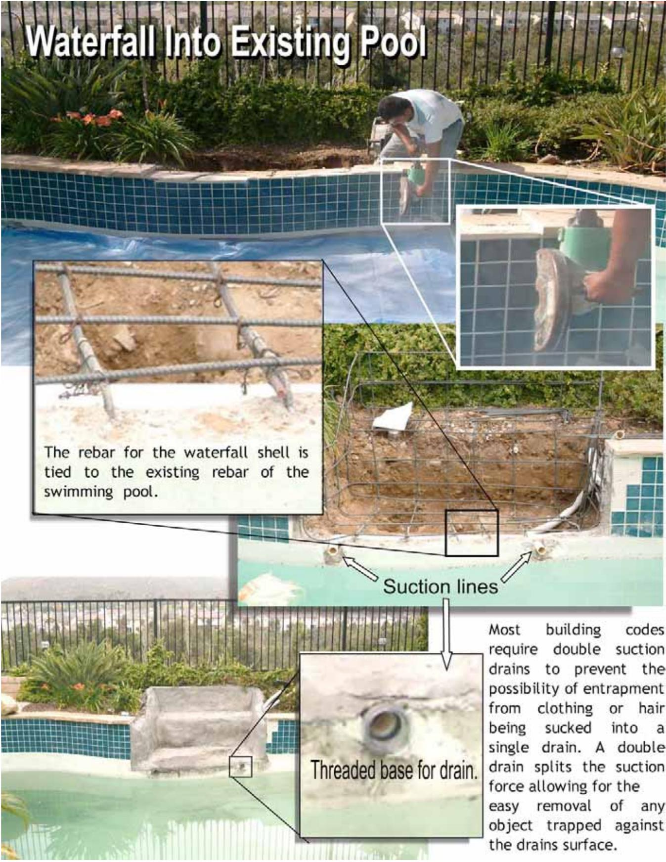
The rebar for the waterfall shell is tied to the existing rebar of the swimming pool.
