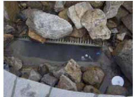
Collection basin containing the anti-vortex drain and AquaFill electronic auto level float control system.
