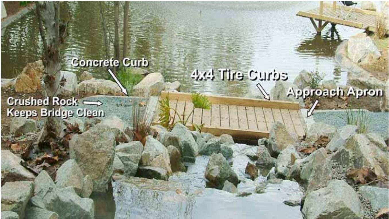
Wooden bridges should not rest in the dirt on either side, but rather supported by a concrete footing or notched apron as shown below. This footing apron was engineered with rebar reinforcement since this bridge supports golf cart traffic.
